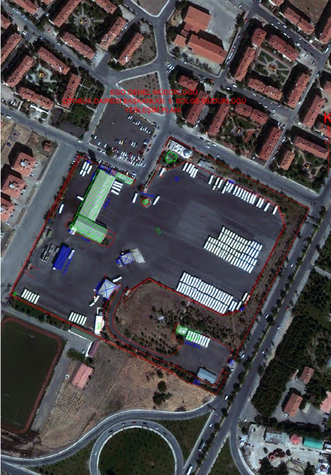
Photo 1.5 Satellite image of the depot in Sincan-Etimesgut (No.5)
